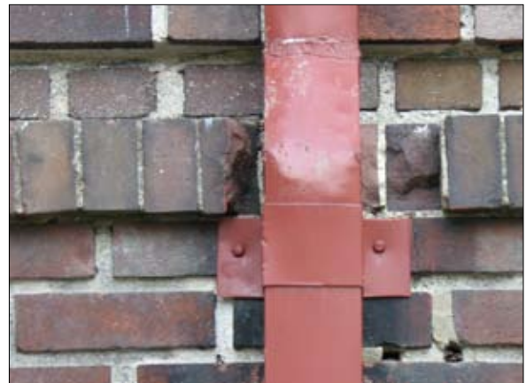
Repair masonry around downspout. Match materials.
