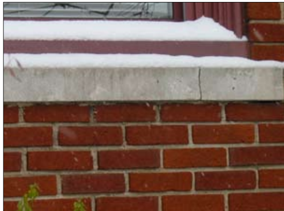
Repair stone sills as needed to match existing material.
