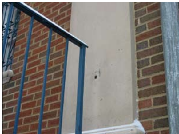
Remove abandoned fasteners, screws, brackets.
