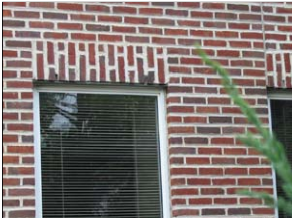
Mortar joints mismatched in size, color, and texture.
