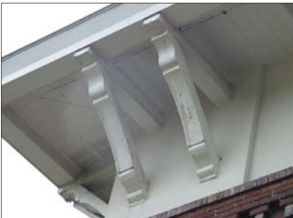
Scrape, prime and paint cornice and trim as needed
