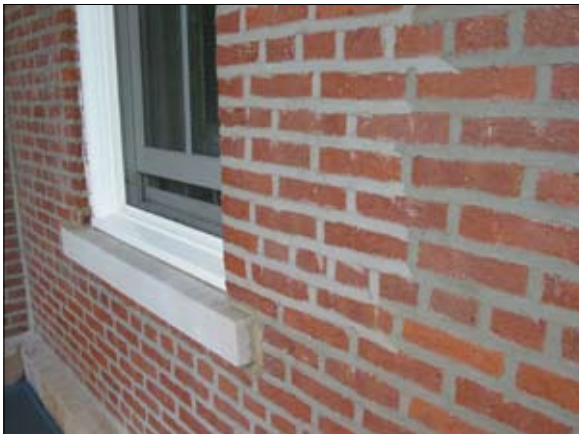
Mortar mismatch. Match color and texture.
