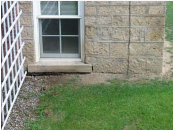
Keep dampness away from foundations.
