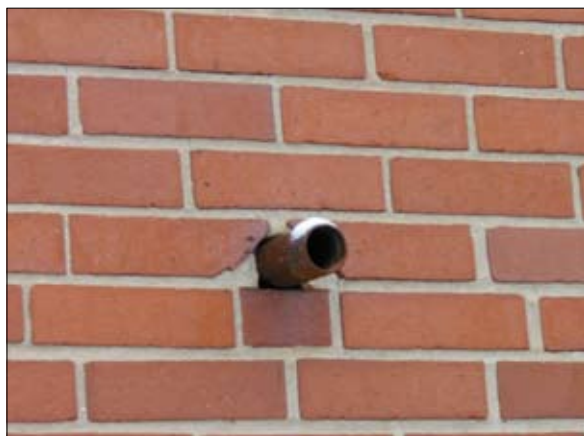
Seal penetrations through masonry.
