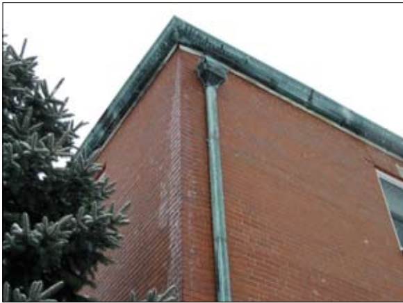
Check eave tubes and gutters for damage.
