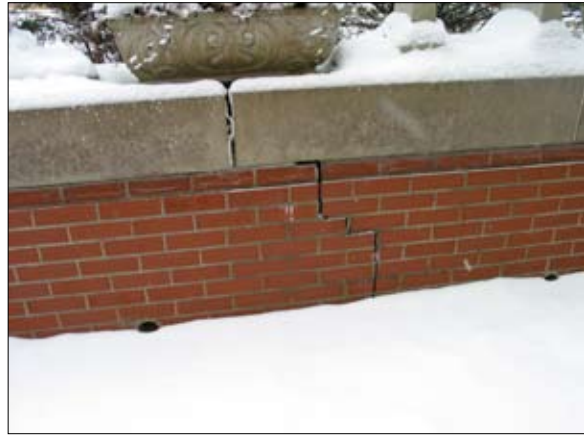
Determine cause of movement. Repair masonry.
