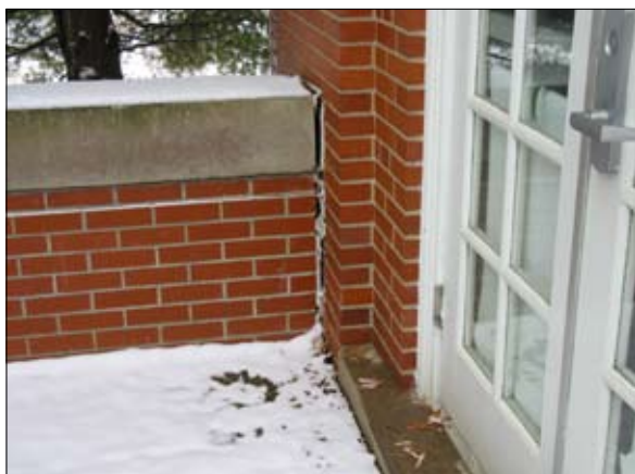
Determine cause of movement. Repair masonry.
