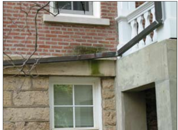
Keep water and dampness off of masonry.
