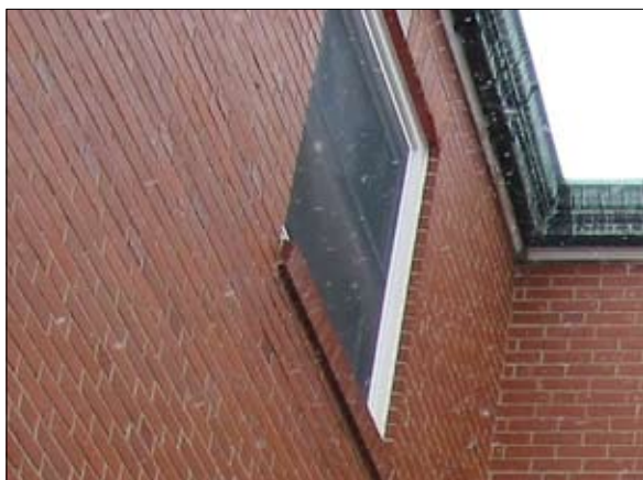
Repoint masonry as needed. Match color and texture.
