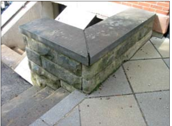
Repair masonry joints as needed.
