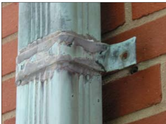
Secure downspouts back to mortar joint.
