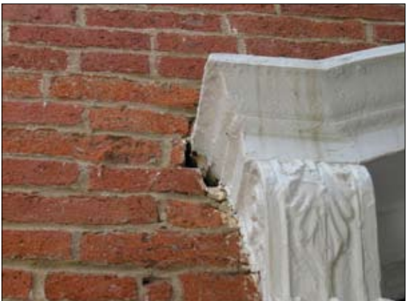
Repair masonry joints as needed.
