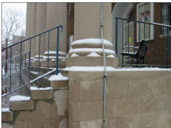
Repair masonry stone with matching color and texture.
