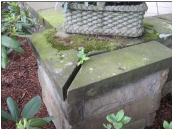
Repair stone caps, matching color and texture.
