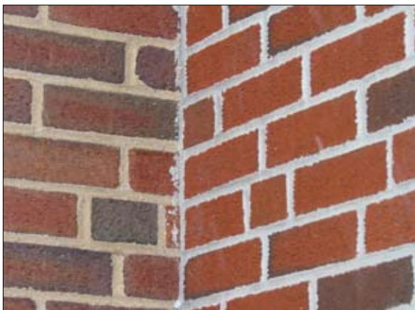
Improper repair. Mortar color and texture mismatch.
