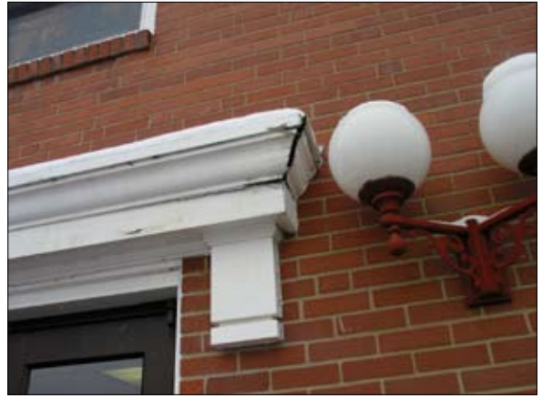
Repair and repaint trim as needed.
