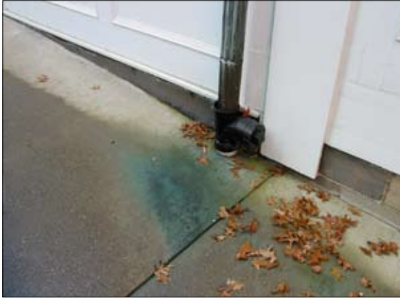
Keep moisture away from foundations, check downspouts
