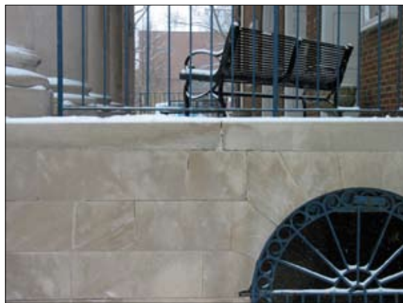
Repoint masonry stone with matching color and texture.
