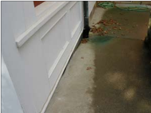
Keep moisture away from foundations, check downspouts
